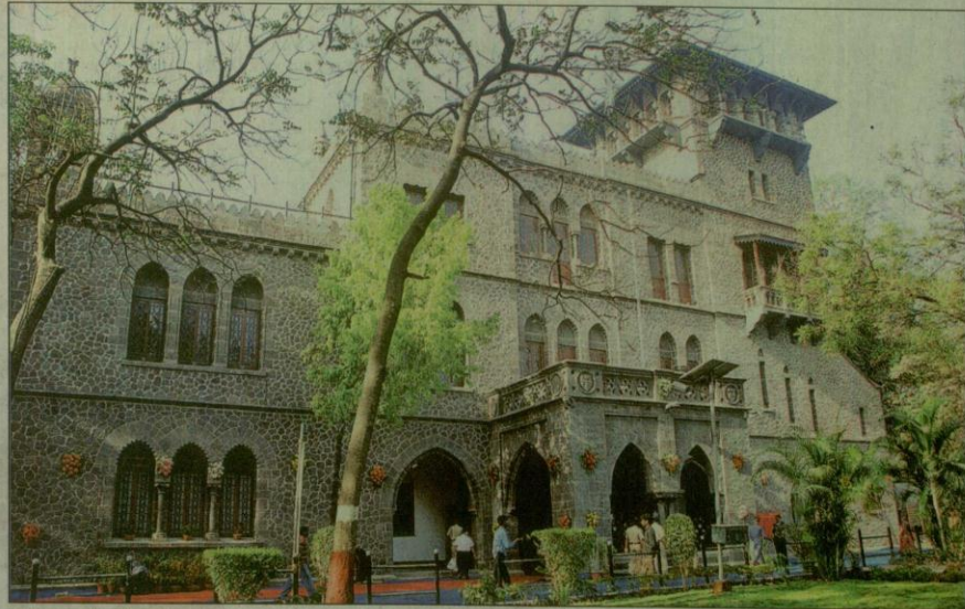
■ The main building of the College of Engineering.
